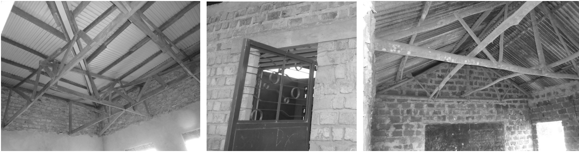
Figure 3a: Inefficient timber roof truss intersection; Figure 3b: metal door and transom; and Figure 3c: truss condition with local site-hewn timber. (Esteban, W. May 2010)
